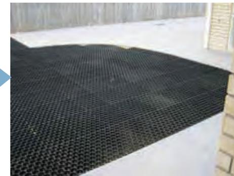
2. JakMats laid using interlocking mechanism
