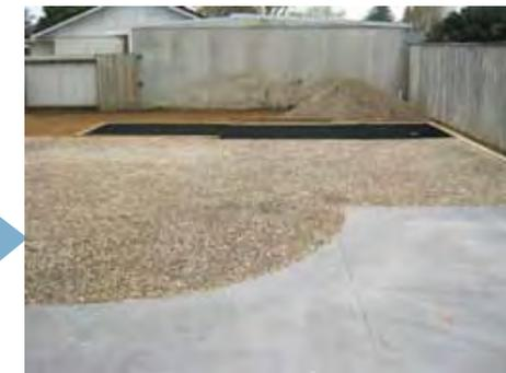
4. P-gravel compact into the honeycomb cells
